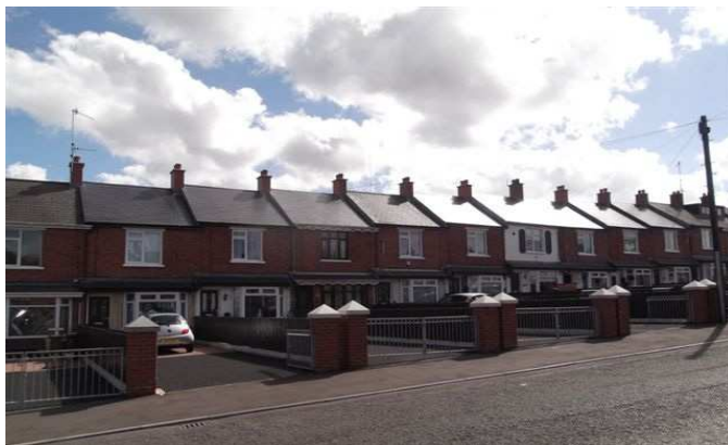
Group Repair scheme Belfast
